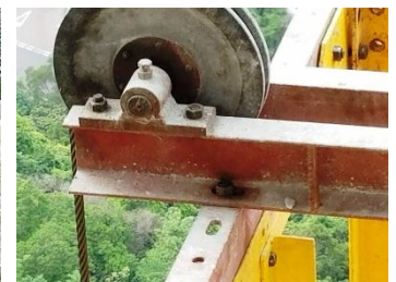
Close-up view of a pulley and supporting members
