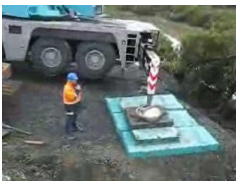
Truck-mounted crane tipping caused by unfirmed ground [Source: Internet]
