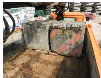
Concrete blocks on truck
