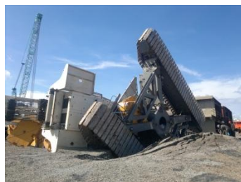
Crawler-mounted crane tipping caused by unfirmed ground [Source: Internet]
