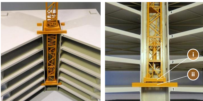
Tower crane mast supported by two sets of support (should be three sets)
