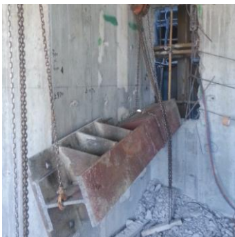
Installation of steel bracket member
