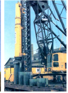
Double-acting hydraulic hammer
