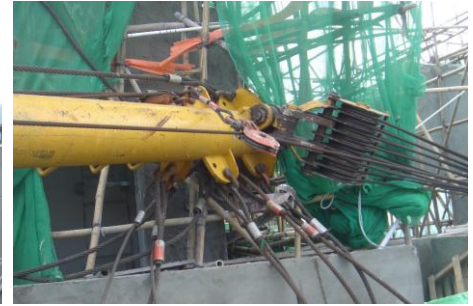
King post top end (with tie-back cables and pulley system for the lifting boom)
