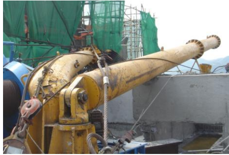
Failed king post (probably initiated by excessive base movement)
