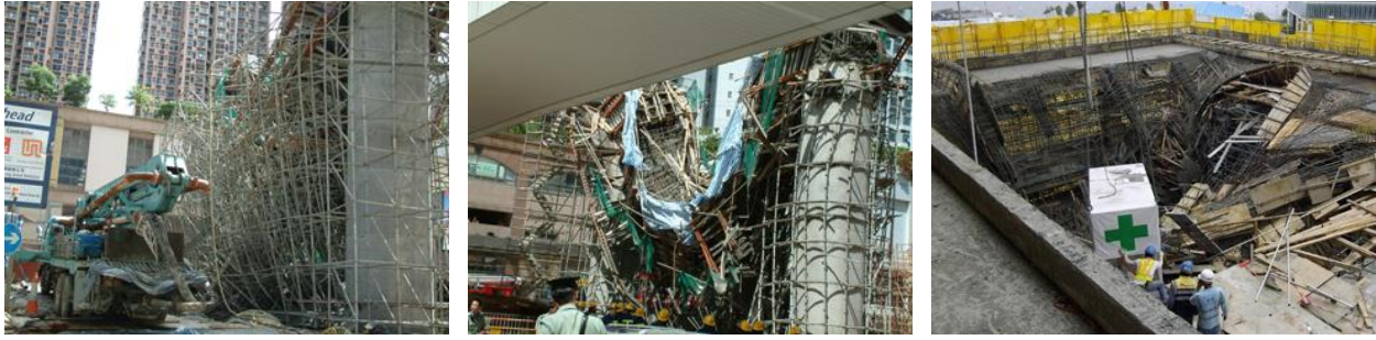
Images of falsework collapse during construction. It was reported that missing cross-bracing was the key reasons for the failure noted.
