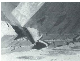
Brittle fracture at steel plates
