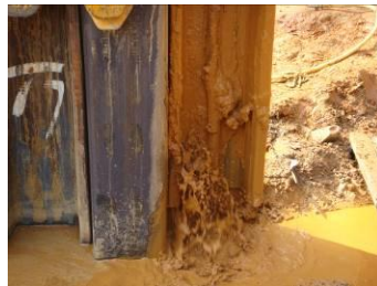
A high pressure flexible hose and water nozzle engaged in the jet lock
