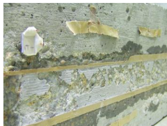
Debonding failure between FRP and concrete substrate
