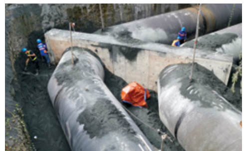
管道安裝包括兩根內徑為 2.5 米的鋼管，分別連接輸水隧道 3 號和輸水隧道 2 號。 Pipework installation consists of two 2.5 m internal diameter steel pipes that are connected to Aqueduct 3 and Aqueduct 2.
