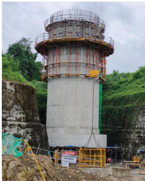
隧道鑽挖機被拆除後，進水口結構的建造已經恢復，預計於 2022 年 2 月竣工。竣工後，該結構的總高度將為 34 米。 Following the TBM removal, the construction of the intake structure has resumed and is targeted for completion in February 2022. Upon completion, the total height of the structure will be 34m.
