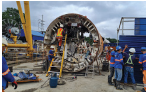
隧道鑽挖機部件的清潔和修復工作。 Cleaning and restoration work on TBM components.
