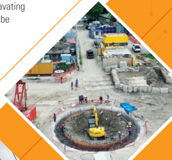
豎井通道施工 Construction Access Shaft
