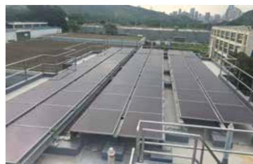
屋宇天台裝設太陽能板，每年節省逾一成耗電量。 Photovoltaic panels on the roof of the building can reduce electricity consumption by 10% a year.
