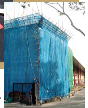
體育大樓的部份結構需要拆卸 Demolition of existing structures at the Sports Complex
