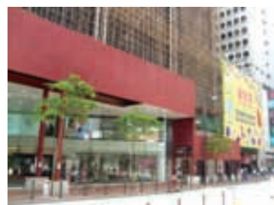
皇室堡改建及翻新工程。 Alteration and addition works at Windsor House.
