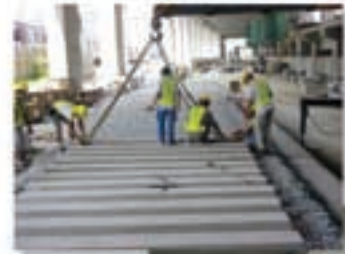
放置道碴及安裝預製石枕承托道岔 Lay ballast and place ties using hydraulic spreader beam for crossover
