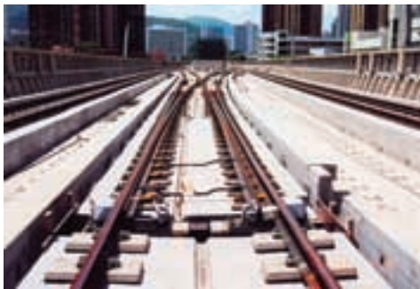
靜音浮板道岔 Floating low vibration turnout
