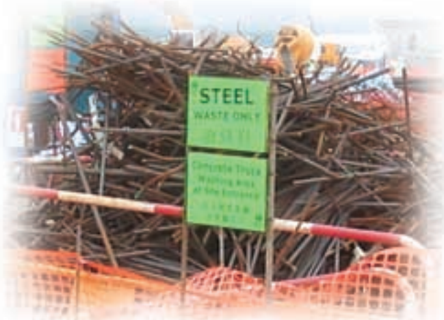
地盤廢物分類 On-site waste segregation
