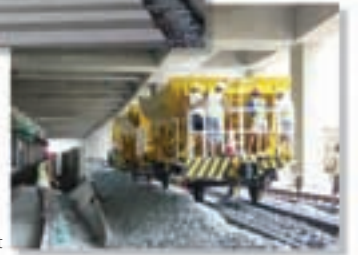
放置面層石碴 Spreading top ballast
