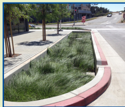
1: Bulb Outs and Curb Extensions
