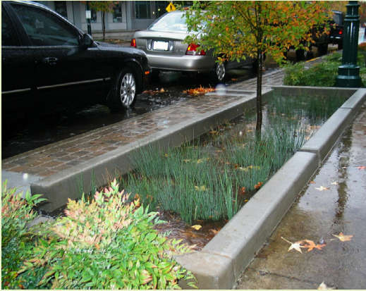
Bioretention treating runoff from the adjacent street during a storm.
