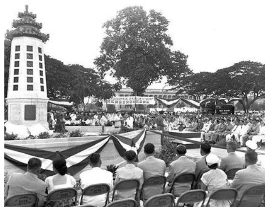
Unveiling of national war hero Major General Lim Bo Seng Memorial by Commander-in-Chief, Far East Land Forces, Sir Charles Falkland Loewen, at the Esplanade Park in 1954. The unique bronze pagoda with four bronze lions was designed by architect Ng Keng Siang and was gazetted as a National Monument in 2010, collectively with The Cenotaph, a war memorial that honours the heroes who fought and died during World Wars I and II, and the Tan Kim Seng Fountain. 29/06/1954. Source: Ministry of Information and the Arts Collection, courtesy of National Archives of Singapore (Media - Image No:19980001068 – 0013)
