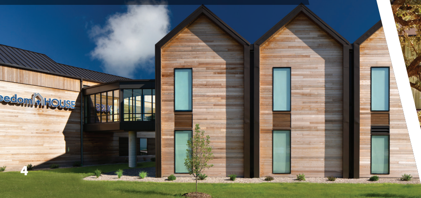
Freedom House, Type V-B, Light-frame/concrete hybrid 140,571 board feet. Courtesy: Tricia Shay Photography
