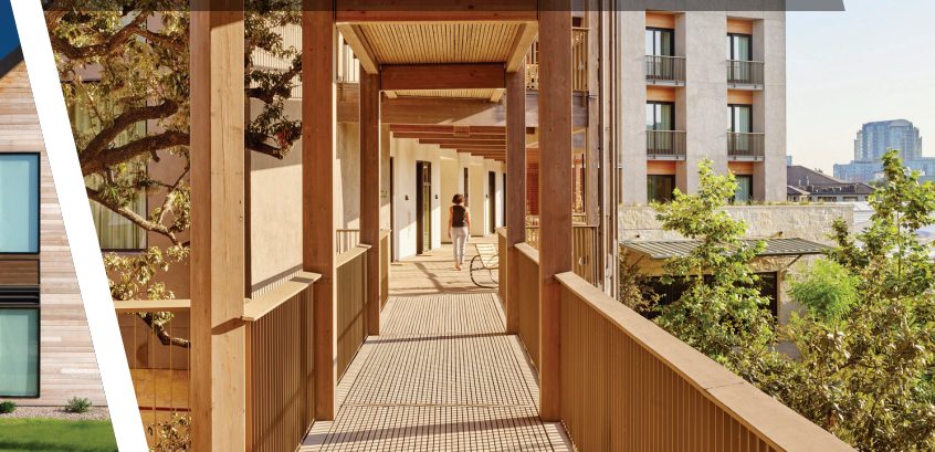
Hotel Magdalena, Type III-B, DLT/light-frame hybrid, three buildings, four stories, 1,140,000 board feet. Courtesy: Casey Dunn
