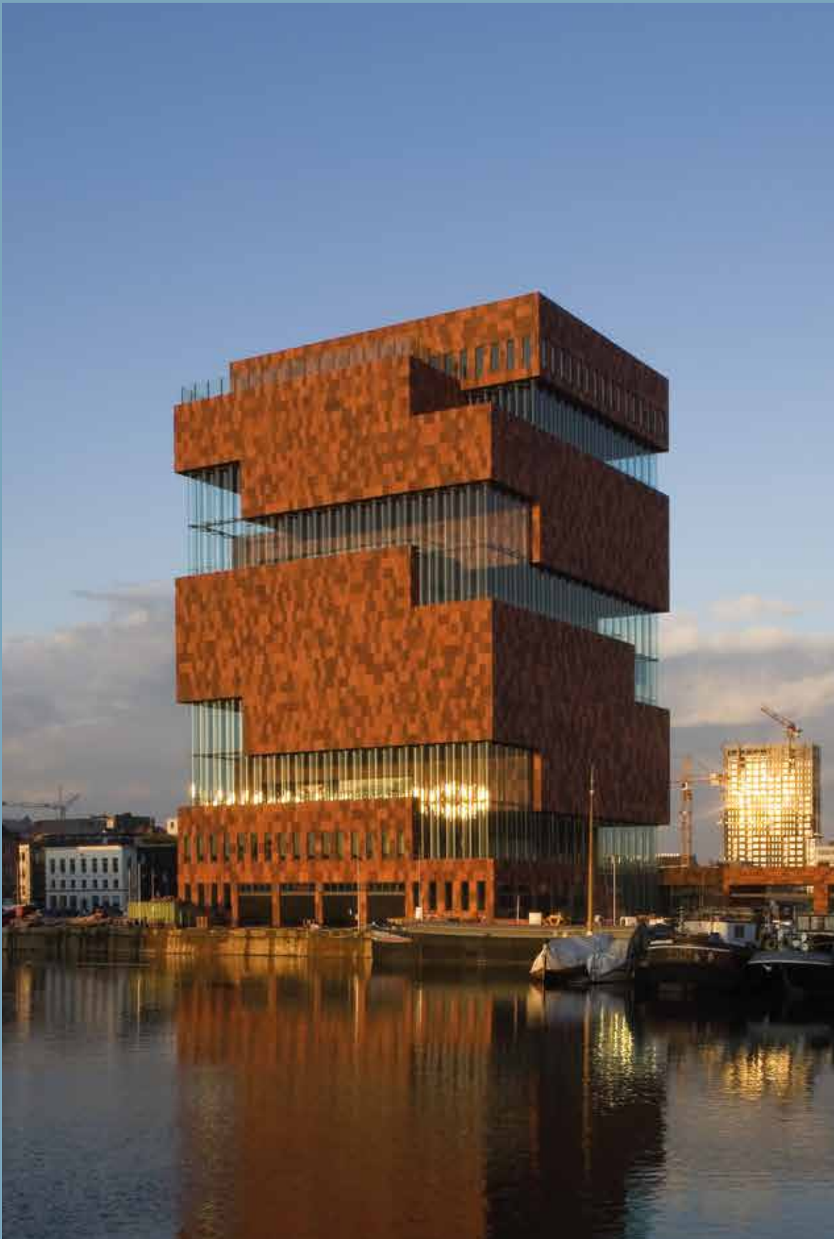
An ambitious and international project: the pavilion of the new Museum aan de Stroom (River Museum) in Antwerp, heated and conditioned with Robur technology. Credits: MAS - City of Antwerp, Sarah Blee
