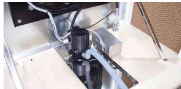
Figure 5.2 Recirculation pump and water distribution system
