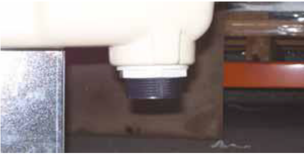
Figure 5.4 Water drain device
