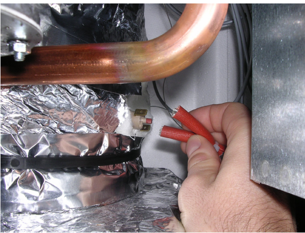
Figure 9.4 Inspection at generator limit thermostat - Detail of thermostat
