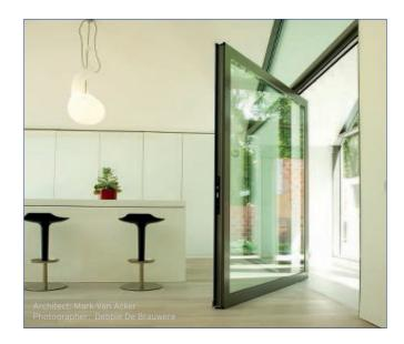
**STYLISH PIVOT DOORS.** A unique and elegant option yielding wider single door leafs than a traditional single panel door. With a hinge mechanism within the floor and header, these doors utilize a pivot motion to open with a clear opening typically 2/3 of the door leaf. With a flush threshold, these doors are ideal for interior applications or covered entry ways.
