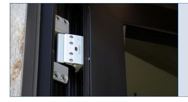
**OPTIONAL CONCEALED HINGES.** Every swing door we build is designed to fit your project perfectly. When you have a Reynaers swing door installed into your home, it will operate flawlessly every time you use it. Our CONCEALED HINGES, available on CS 77 only, are not only aesthetically remarkable, but are adjustable on all three axis to ensure impeccable operation. The offset design yields a wider clear opening than a door of similar size with barrel or surface mounted hinges.
