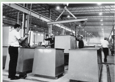
Operating a 30-ton overhead crane to position loading tanks onto the test assembly.
