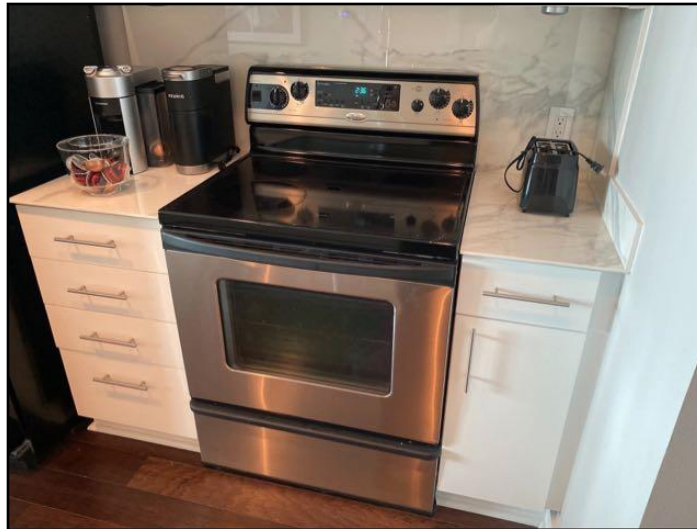
15. Anti-tip device missing/defective
