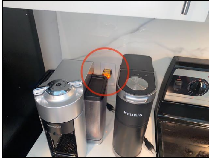
2. Test faulty on GFCI (Ground Fault Circuit...
