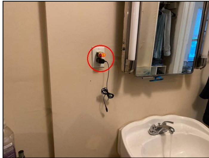
20. Test faulty on GFCI (Ground Fault Circuit...
