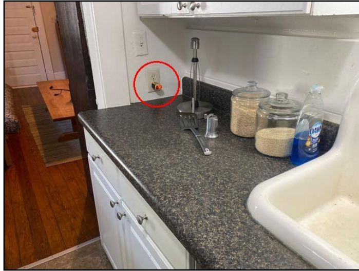
21. No GFCI/GFI (Ground Fault Circuit...
