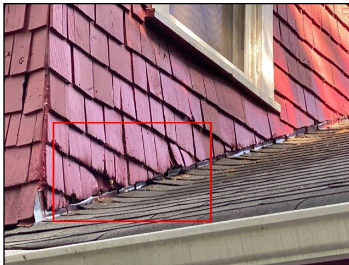
9. Rot/Insect damage
