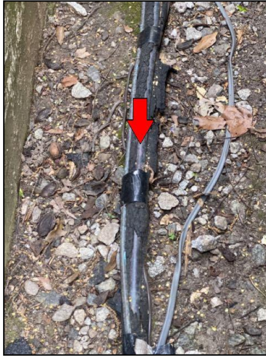
27. Missing Insulation
