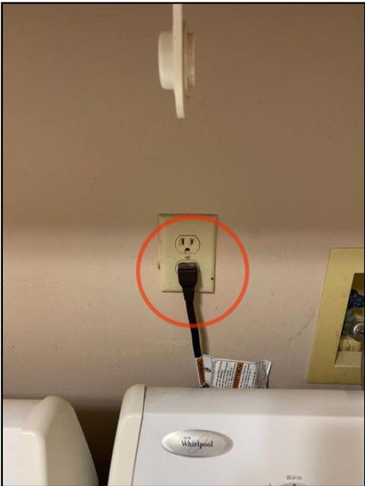
62. No GFCI/GFI (Ground Fault Circuit...
