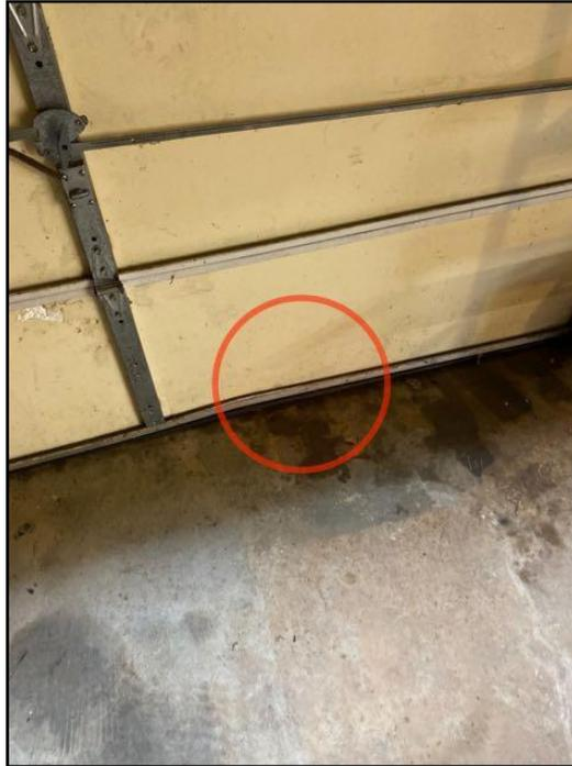
44. *Vehicle Door is Dented/Damaged*
