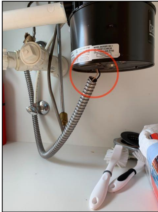
50. Wiring exposed or loose
