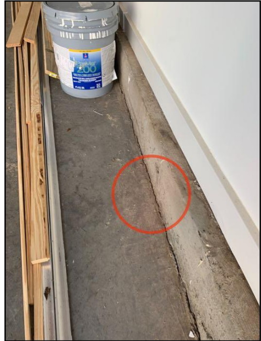
12. Cracks in Floor
