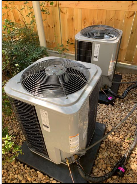
30. Air Source Heat Pump
