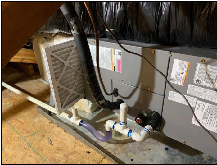
25. Heat pump - Electric (Interior Unit) 20-25...
