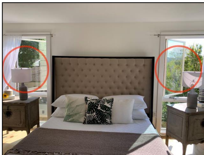
42. Weather Stripping Needed-Master bedroom
