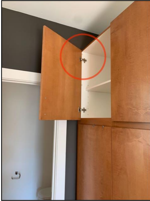
45. Pieces missing or loose
