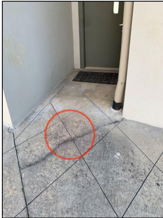
10. Cracked or Damaged Surfaces
