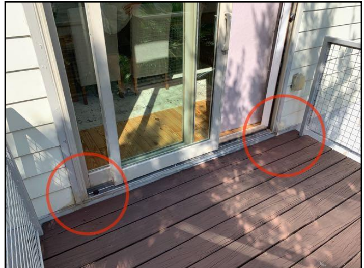
8. Rot/Insect damage
