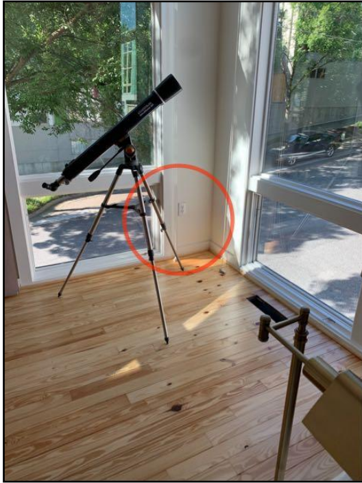
16. Loose Receptacles-Living room
