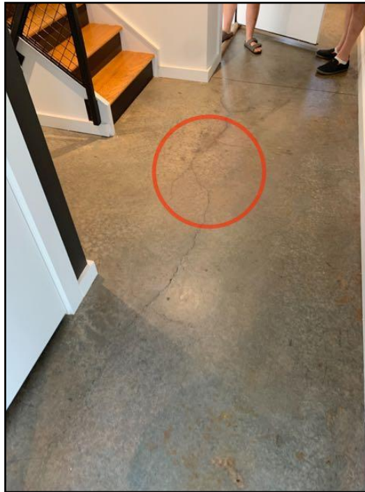
40. Concrete Cracked-Basement
