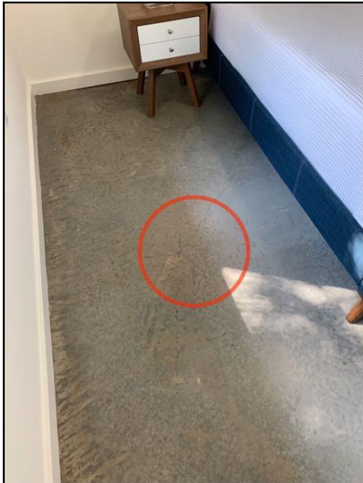
38. Concrete Cracked-Basement
