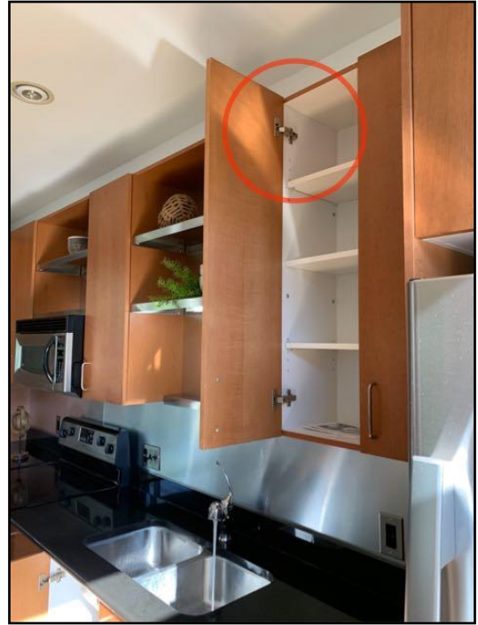
46. Pieces missing or loose
