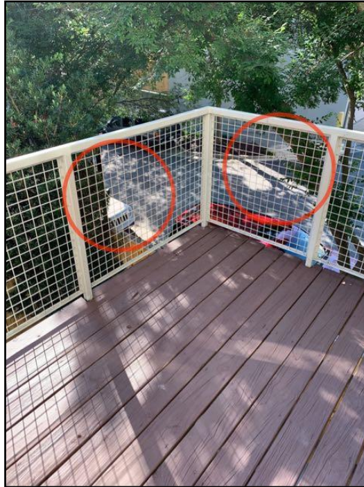
9. Balusters/spindles climbable
