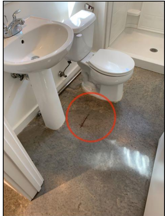
39. Concrete Cracked-Basement
