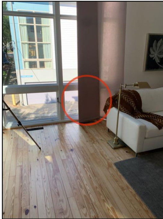
41. Windows Painted Shut
