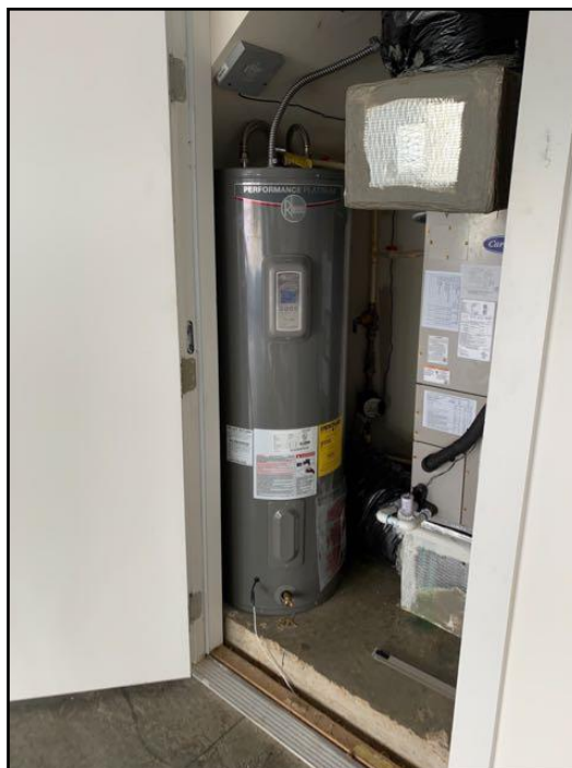
36. Conventional (Tank) Electric Fuel - 8-12...
