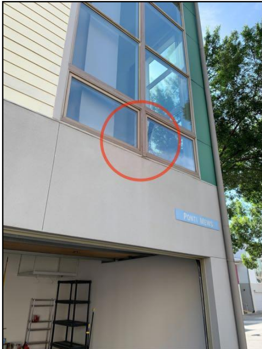
7. Rot/repair and seal
