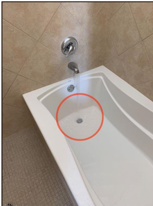
34. Drain stop ineffective
