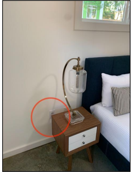
17. Loose Receptacles-Basement bedroom
