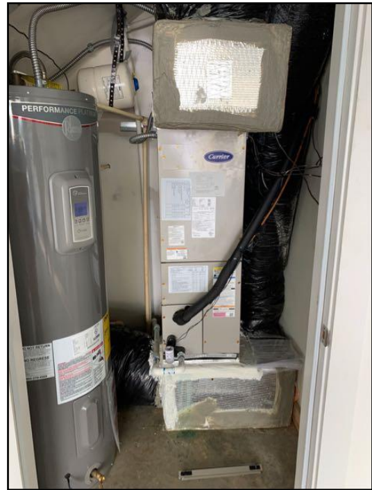
26. Heat pump - Electric (Interior Unit) 20-25...
