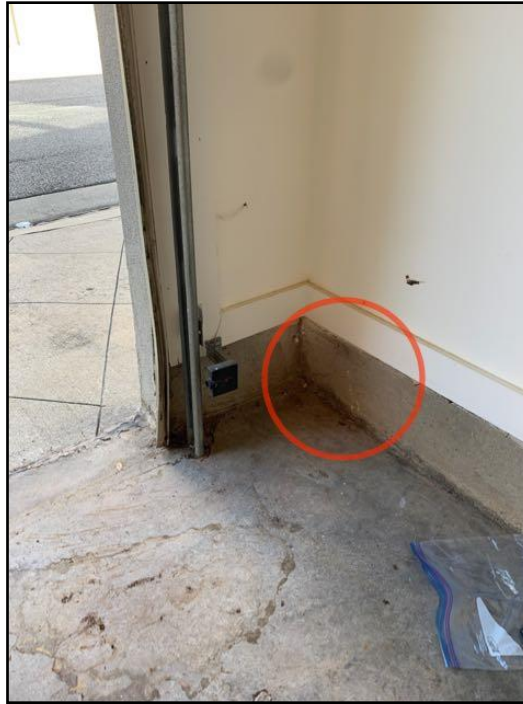
14. Typical minor cracks/settling
