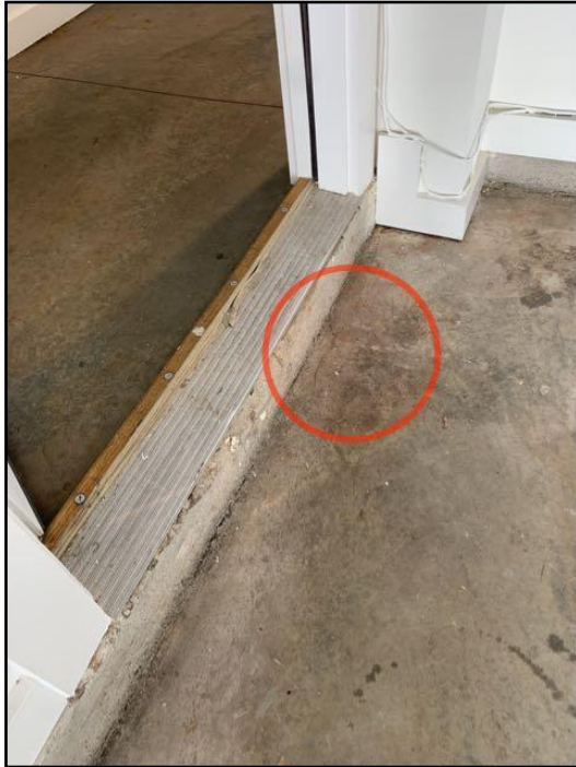
11. Cracks in Floor
