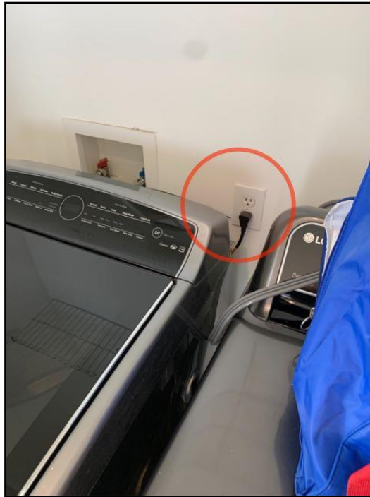
15. No GFCI/GFI (Ground Fault Circuit...
