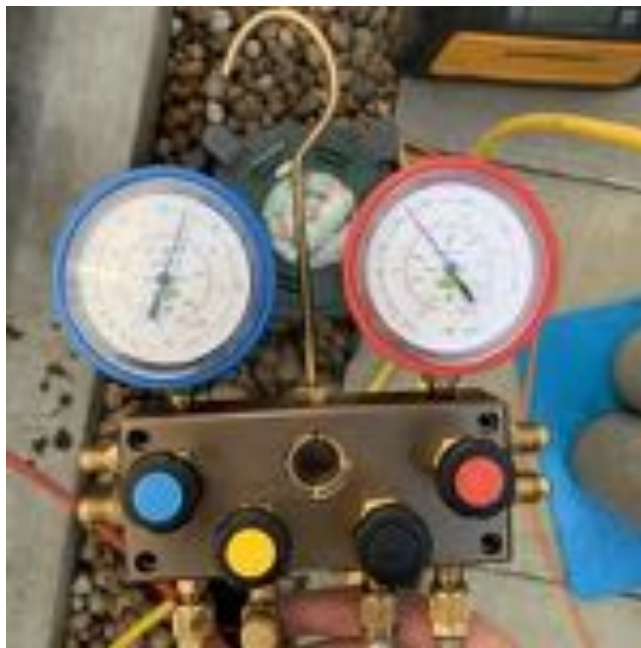
Pressure test readings
